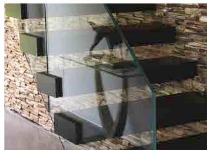
GLASS WITH CONCEALED FIXINGS Timber covers fitted on to the glass balustrade to conceal the button fixings.
