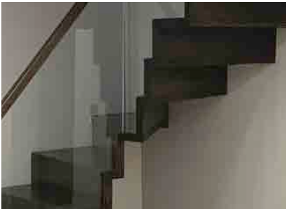
90 DEGREES - WINDERS A 90° turn toward the next level, creating an 'L Shape' with a seamless transition.
