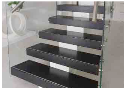
FLARED Increasing the width of the bottom treads gives a slight curve to the stairs.
