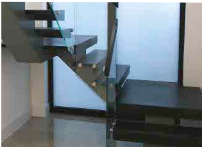
180 DEGREES - 2 QUARTER LANDINGS Two flat quarter landings create a 'U shape' and break the stairs into small sections.
