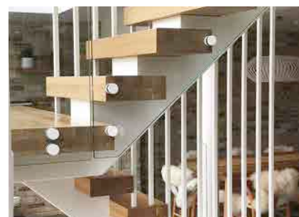
SQUARE SPINDLES Square spindles for an enclosed feel, fixed to the handrail and stair treads.
