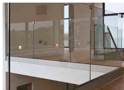
GLASS IN U-CHANNEL An invisible look with clean lines, the glass can be fixed into a U-Channel profile.
