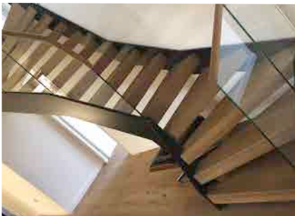
S SHAPE The stair sweeps one way and then the other using winders to create an 'S Shape'.
