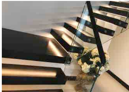
90 DEGREES - QUARTER LANDING An 'L Shape' bend is achieved by adding a quarter landing at the transition point.
