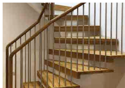
ROUND SPINDLES A classic feel, stainless steel spindles are fixed to the handrail and stair treads.
