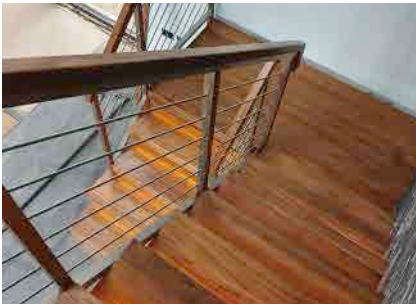
180 DEGREES - HALF LANDING A flat platform, allowing the stairs to undergo a half turn.
