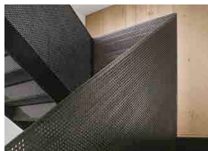
STEEL SHEET BALUSTRADE Perforated steel sheets, typically 4-6mm thickness, or bespoke cut designs.
